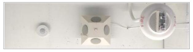
Figure 20, Shows the ceiling where the sound masking system is installed in ASID headquarters office. (Source: Architectural Health/Yan Architects LLC, 2019)
