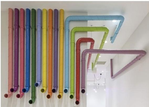
Figure 11, Using color for pipeline classification
